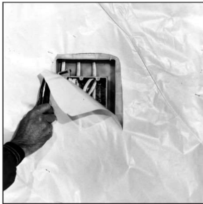
Cut air barrier at center of flanges of LESSCO® Box.
