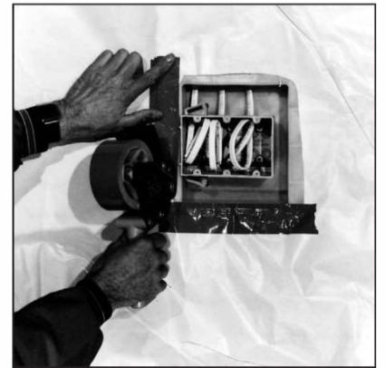
Tape the air barrier to the flanges of the LESSCO® Box
