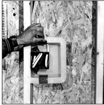
If hinge feature was used, tape openings at top/bottom of LESSCO® Box.
