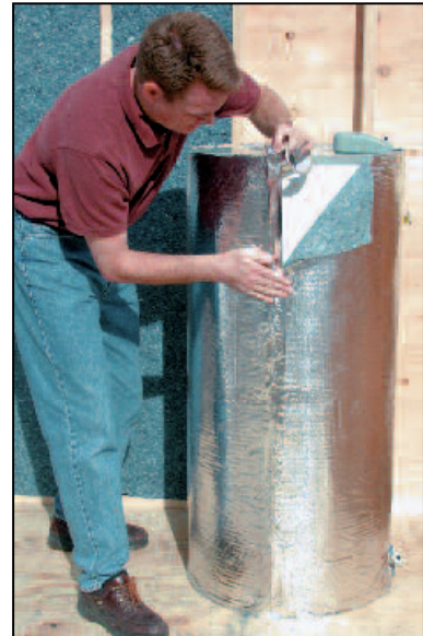
This image is of an installer taping the vertical seam of an electric tank. Note that the jacket goes all the way to the floor, which is not advised on oil or gas water heaters.
